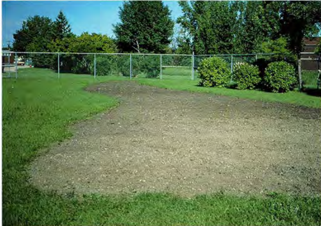
An excellent site preparation at Elmwood High, Winnipeg – spring 1991.
