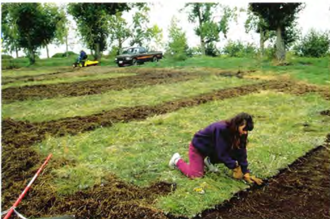
Laying salvaged native sod in Calgary.
