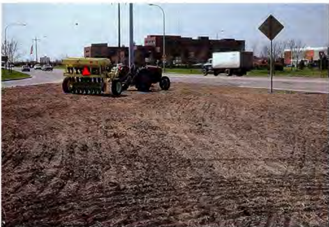
Covering the area twice, with the second pass at right angles to the first will eliminate rows and look more natural.
