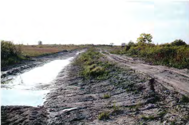
Newly exposed subsoil from construction projects can provide a clean, weed free medium for prairie restoration.
