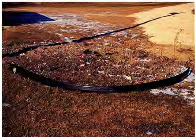
Install a continuous deep lawn edging around all school and backyard plantings to keep out invasive non-native lawn grasses.
