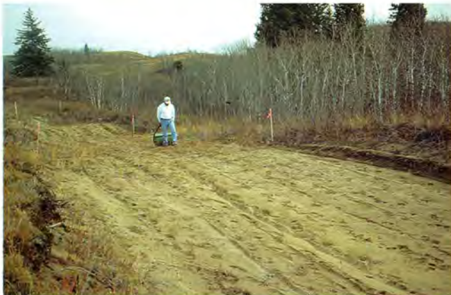
A hand roller here is being used AFTER broadcast seeding.
