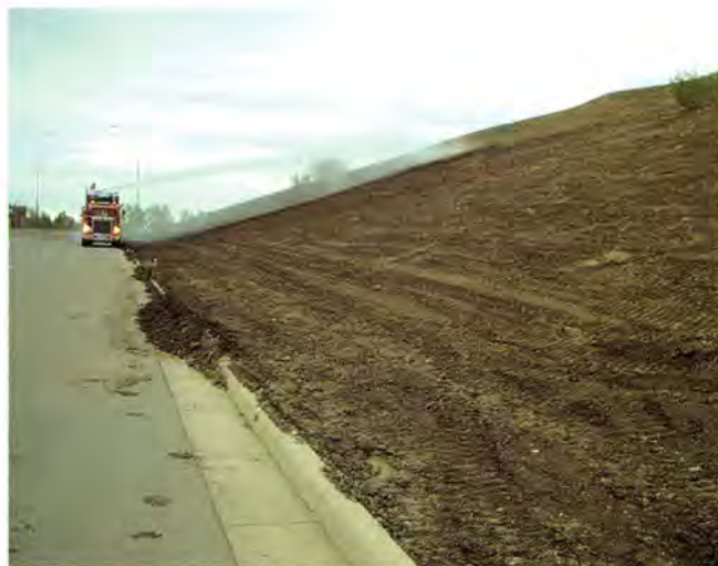
Hydro seeding a prairie restoration on a slope in Calgary.
